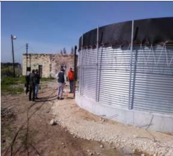
Constructing an about 500 m 3 water tank for the university
