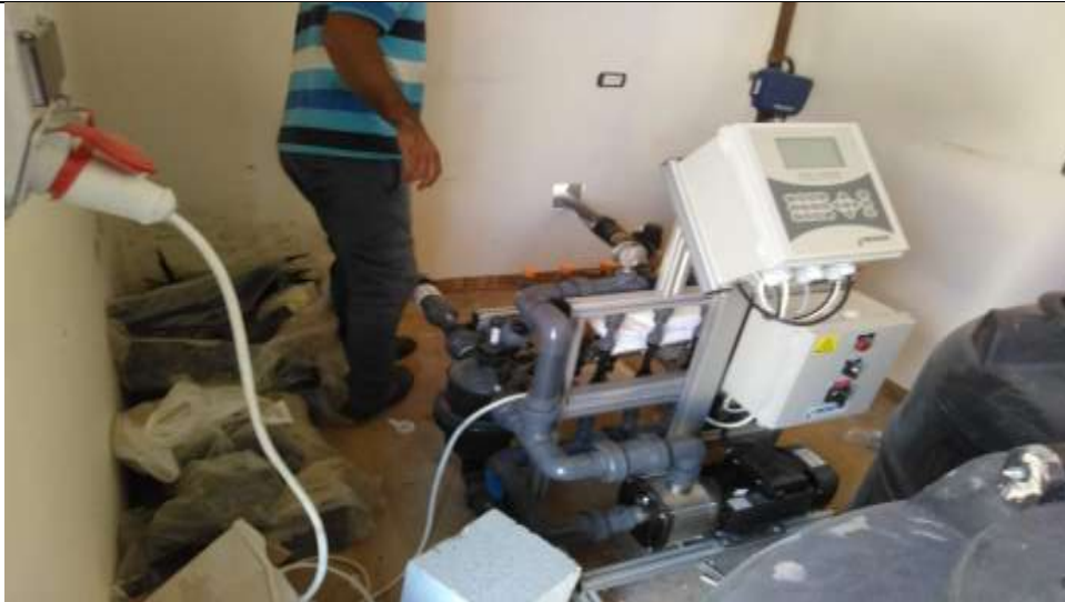
Automatic Irrigation and Fertilization
