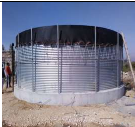
Constructing an about 500 m3 water tank for the university
