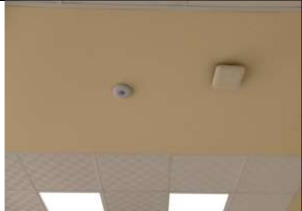
Motion Detector Sensor inside class rooms and corridors
