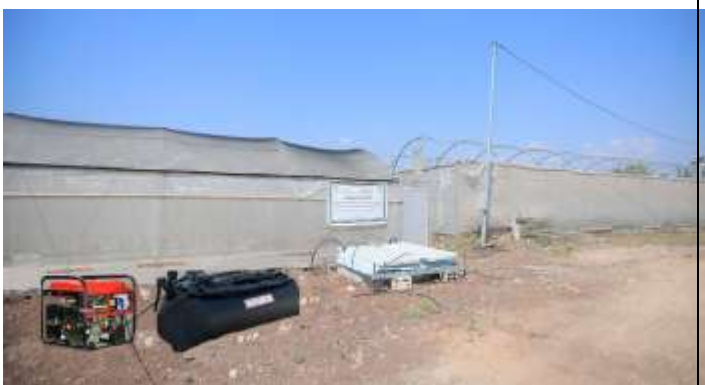
Example of Biogas digester generating biogas to supply a methane engine generator (PTUK – Main campus, Tulkarm, Palestine)
