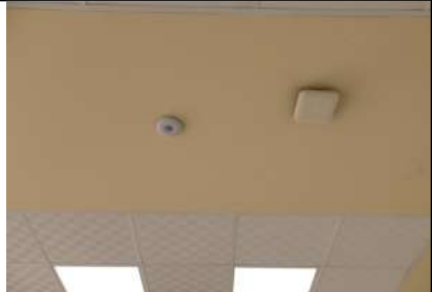
Motion Detector Sensor inside class rooms and corridors
