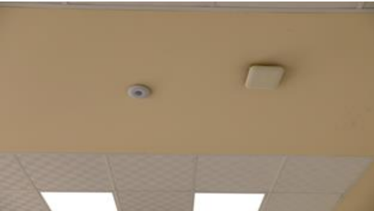
Class rooms with motion detectors to control lighting inside rooms with presence of students
