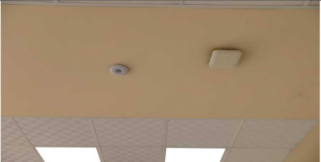
Motion Detector Sensor inside class rooms and corridors
